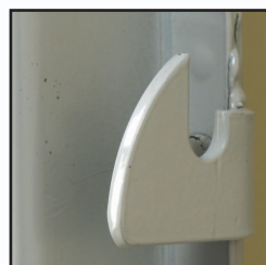
12 gauge latch hook is welded to frame
